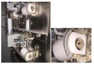
Motor running + Solenoid actuated = Line not visible Motor running + Solenoid not actuatuated = Line visible
